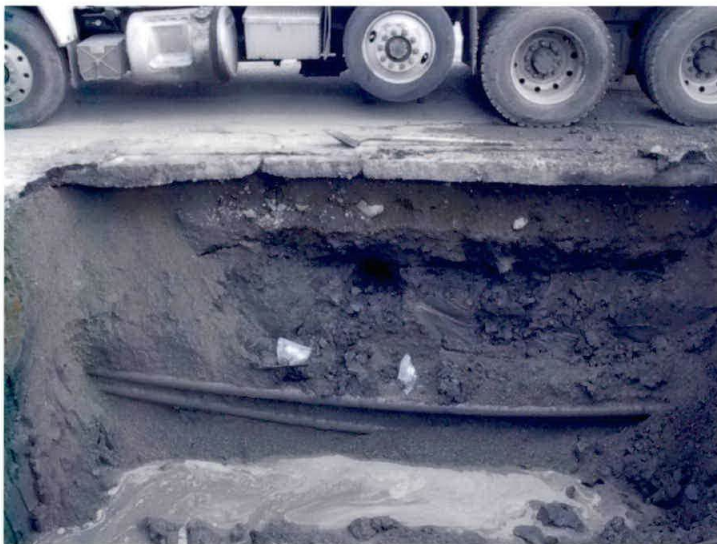
Photo 11. South wall of the excavation, view looking south. Residual concentrations of gasoline, benzene, cPAH, and lead exceeded Method A cleanup levels on this sidewall, beneath Morris Street.
