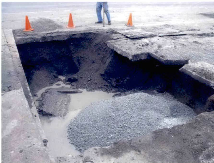
Photo 14. Initial load of backfill material consisting of crushed rock.
