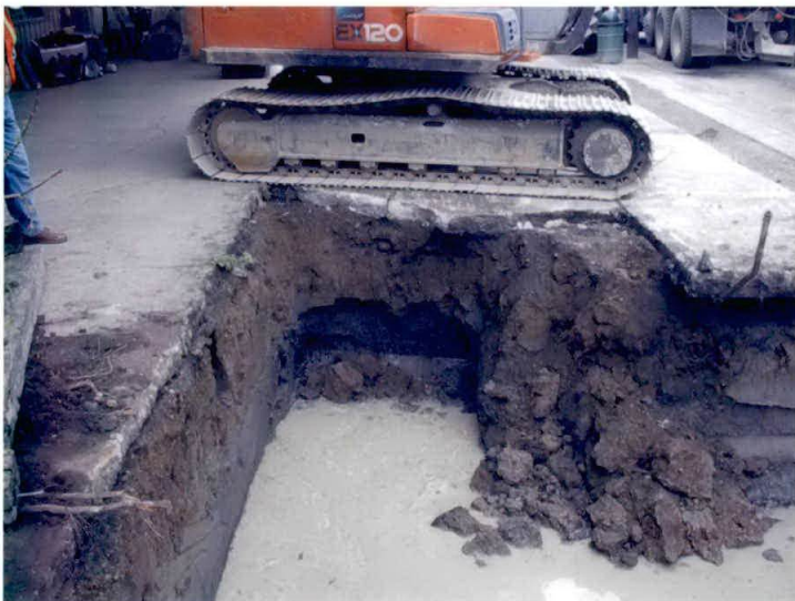
Photo 12. North half of the east sidewall, view looking east. Residual concentrations of gasoline and cPAH exceeded Method A cleanup levels on this part of the sidewall.
