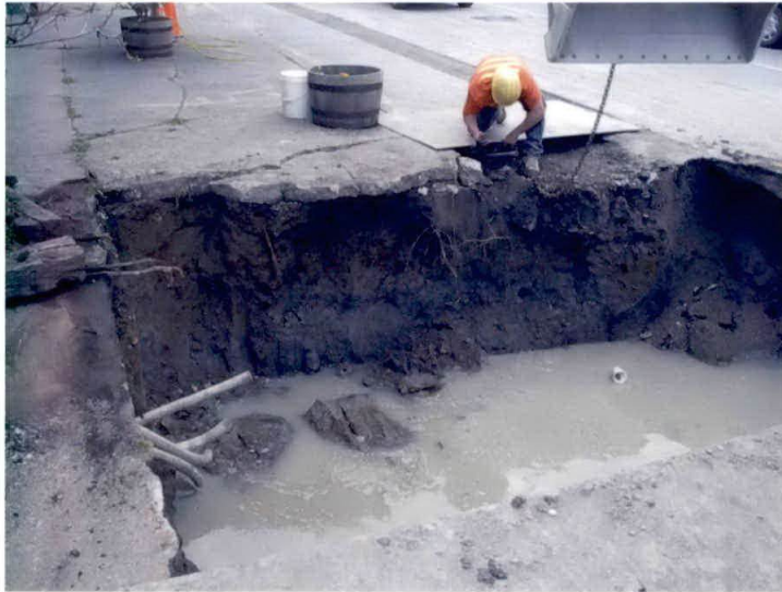
Photo 10. Possible distribution pipe located on the east side of the UST pit, view looking east. The pipe could not be moved with the excavator.
