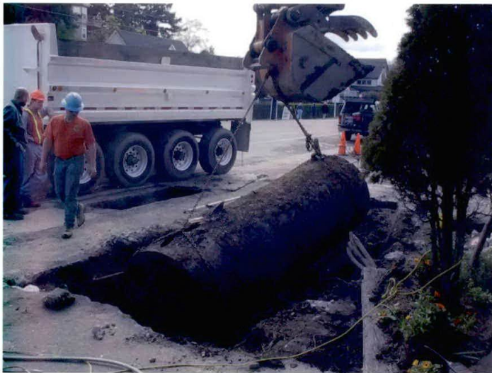
Photo 4. Removal of UST #1. The vent pipes can be seen in the central right part of the photo.
