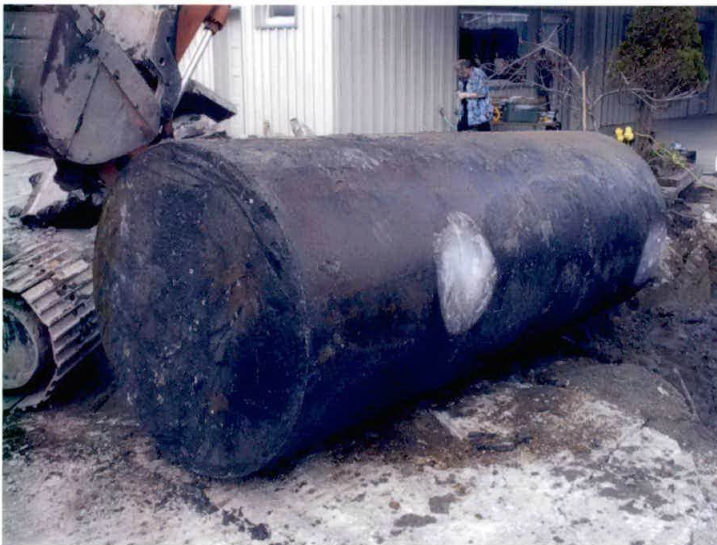
Photo 8: The lower half of the tanks (except UST #4) were observed to be in good condition, with only minor corrosion and pitting and no holes. The lower half of UST #4 had holes.
